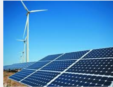
Utilities - Distribution of electric energy for low and medium voltage
